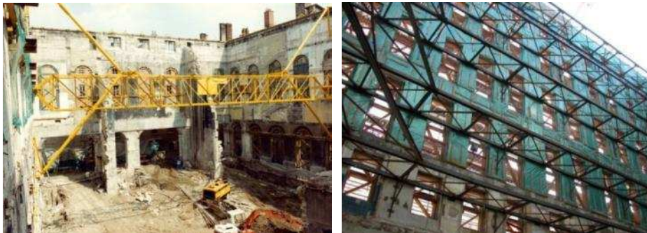
Fig. 3. Renovation bracings strut-type of historic facade walls [4]
