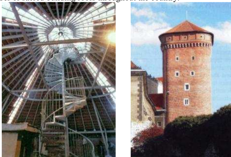
Fig. 7. The horizontal bracings in the steel reconstruction of the Lubranka tower roof on the Wawel (left) and a view of the object after completion of maintenance works (right) photo by P. Stępień [10]
